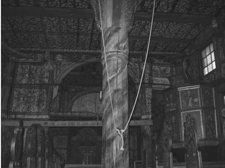
Figure 2.11. The central pillar supporting the roof structure at Uvdal. The ceiling above it is an early modern modification which may contribute to better heat retention, but which prevents any sight of the branching of the rafters away from the “tree trunk.” The early-modern artist who decorated the church may have been aware of the Yggdrasil tradition, for he painted an enveloping and luxuriant spread of leaves and vines on the ceiling and walls of the entire church. The central wooden stave or tree trunk structure used in Norway was paralleled by the central stone pillar design of the round churches on Bornholm in Denmark. Author’s photograph.
