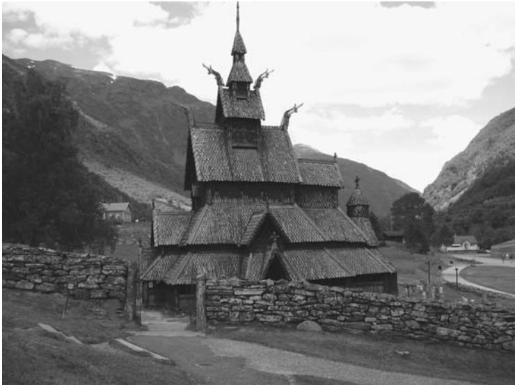
Figure 2.1. The Borgund stave church seen from the southwest. The path leading down to the left ends at the western entrance. On the roofs and walls wooden shingles are everywhere, giving protection from rain and snow. The lower gables end in crosses, but on the upper gables are prominent serpents. The low stone wall encloses the church's graveyard. Author's photograph.
