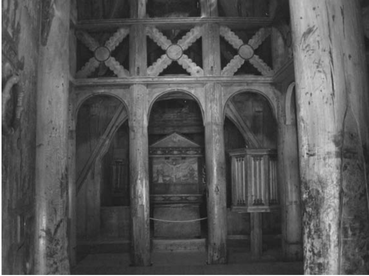
Figure 2.2. Interior view of the east end of the Borgund stave church, showing the wooden staves or pillars, and the fished arches made of knees. Up above are the x-shaped struts (the St. Andrew's crosses) which serve to bind the stave structure together. They are carved with patterns of stylized leaves on branches. The nave is somewhat small but comfortable, as is the sanctuary, but what the church may lack in grand floor space it makes up for in height. Author's photograph.
